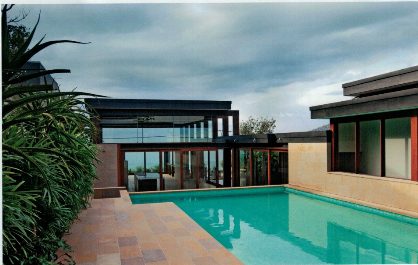
FINALIST PARTNER Shriro Commercial | BUILDER Mardini Constructions | Suite 3, 187 Marion Street LEICHHARDT NSW 2040 PHONE 02 9568 3201 WEBSITE mardiniconstructions.com.au
